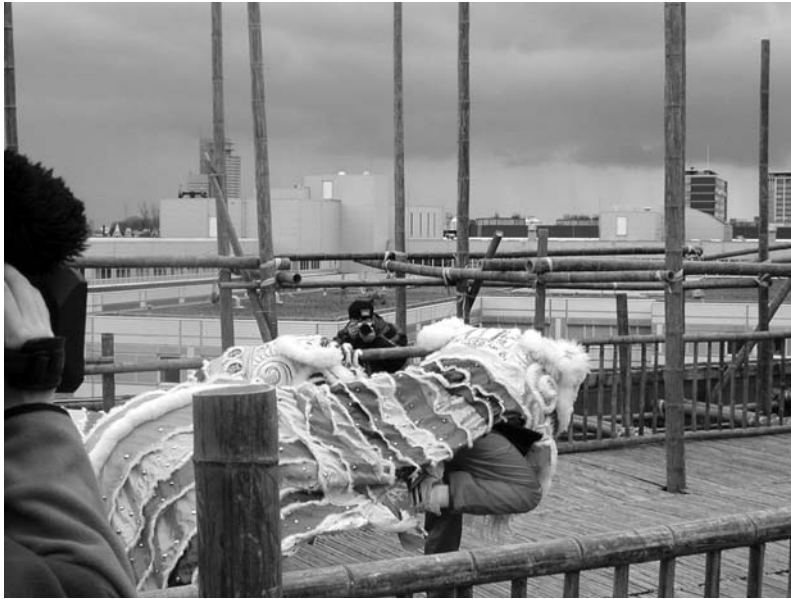
Figure 11.6 Building the bamboo structure: the opening dragon ceremony. (Source: Hulshof Architects.)
